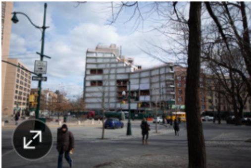
The site, seen here under construction, was for decades home to a gas station. PHOTO: KEVIN HAGEN FOR THE WALL STREET JOURNAL
