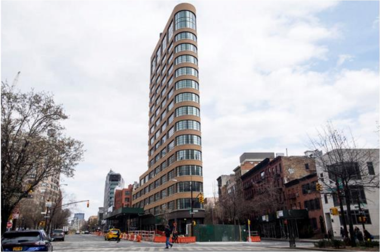
A new corner building at 10 Sullivan Street in the SoHo section of Manhattan.
